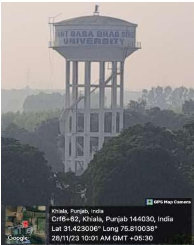
Main Water storage Tank
