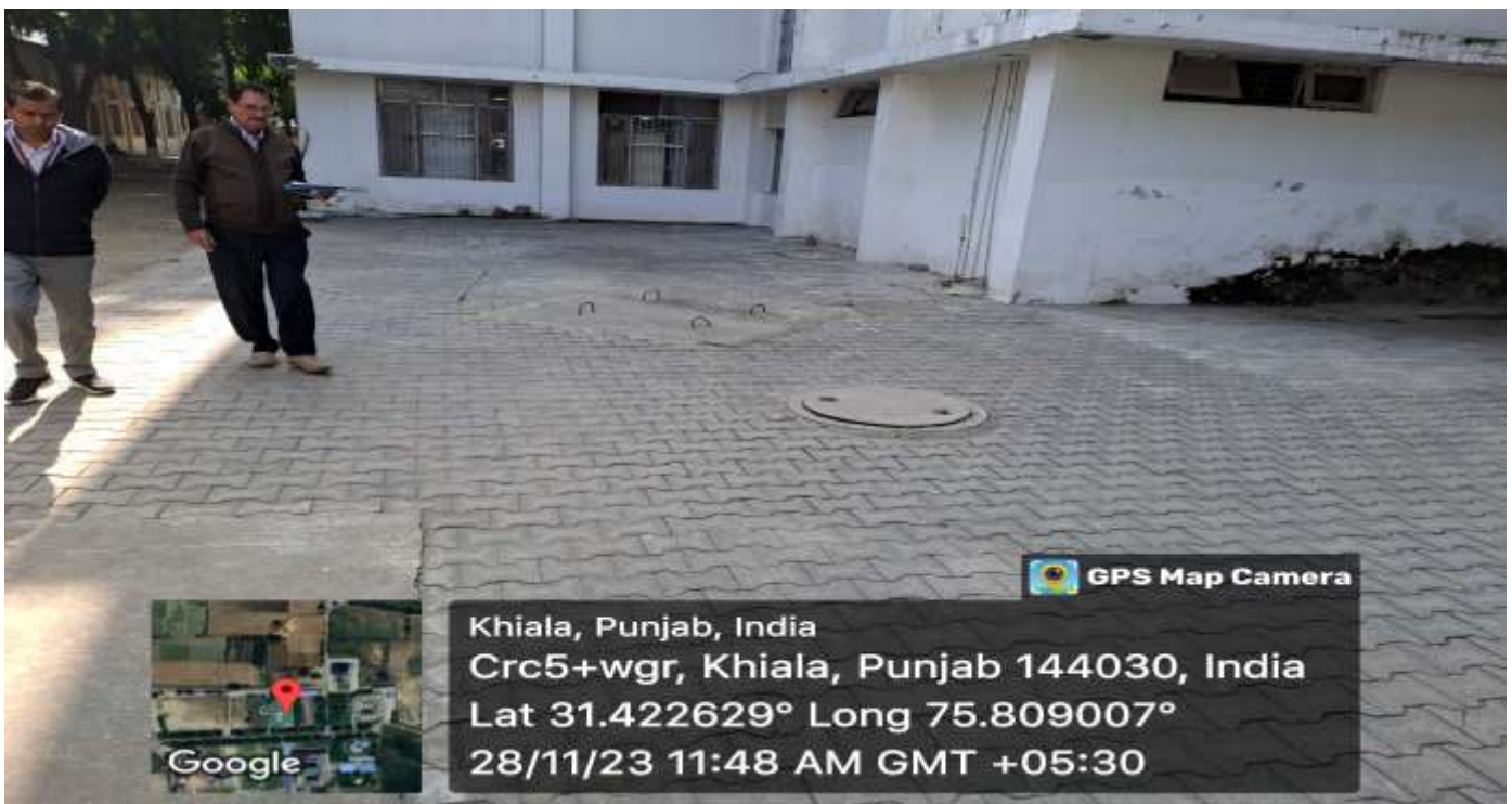
Rainwater Harvesting Tank Near Block 5 at SBBSU Jalandhar
