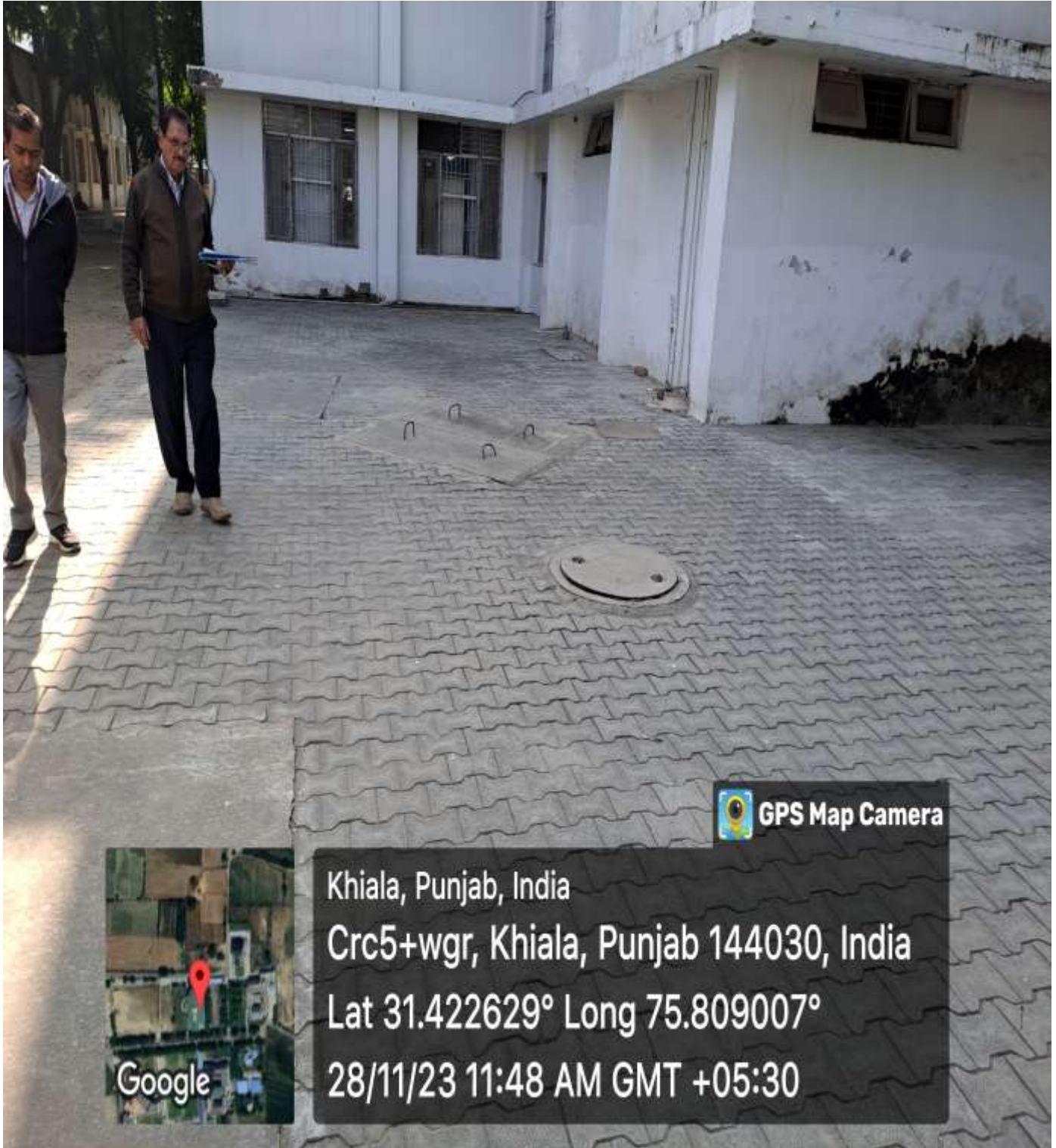
An Underground Rain Water Harvesting Tank in SBBS University Campus.
