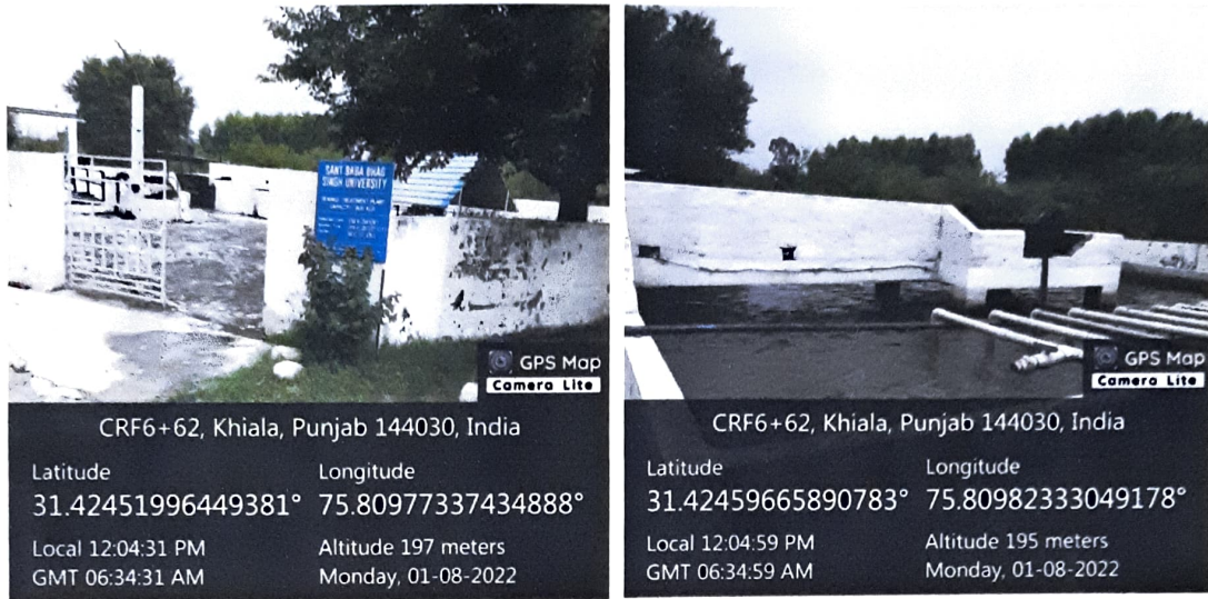
Figure 4 Sewerage Treatment Plant (STP) of capacity 600 KLD
